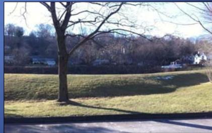
A levee is an earthen structure made of clay or other structural fill material. Examined in cross section, it is a triangle with the top leveled off. The base is commonly 10 times as wide as the height. It can be designed to support pedestrians or even cars.
