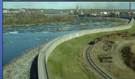
A flood wall is built with concrete and/or steel. It can be built either on top of a levee or in place of a levee. Generally, it is built where there is not enough space for the levee's broad base. One critical difference between levees and floodwalls is that a levee can still provide some flood control function if some erosion or water overtopping occurs, but floodwall failures can be catastrophic.
