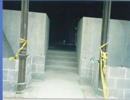
Here are some visual examples of floodproofing. The example on the left includes a waterproof membrane behind the brick wall and the modifications on the right make changes to the entry of a property. When walls are floodproofed, windows, doors, and other openings must also be addressed.
