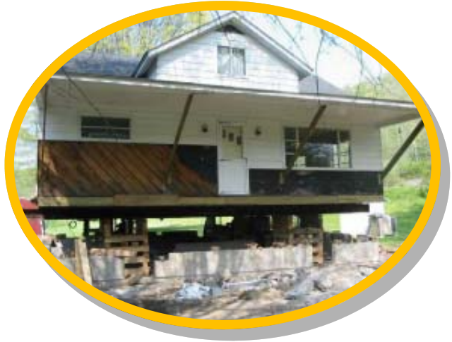
House being raised to construct new elevated foundation.
