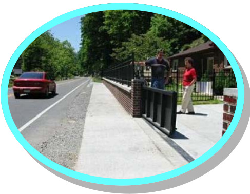
Floodwall that requires opening to be manually closed.
