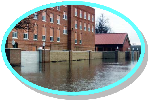
Masonry floodwall with engineered closures.
