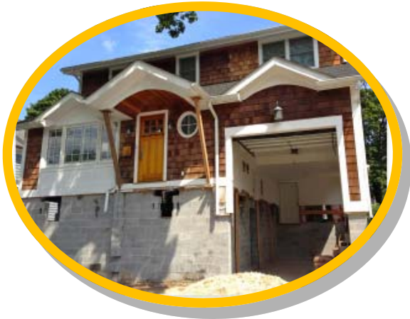
House elevated on extended foundation.
