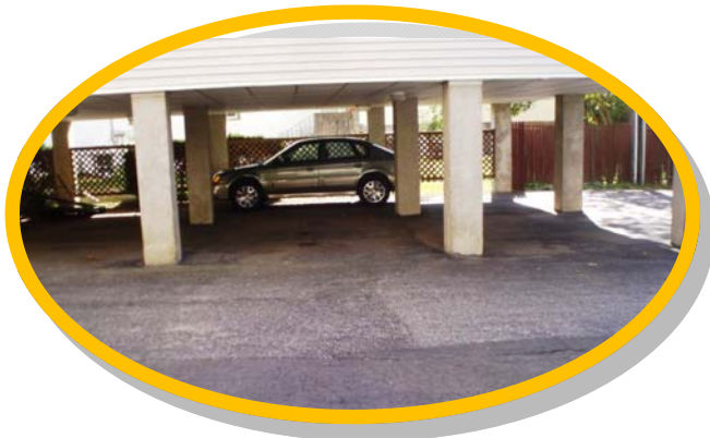
House elevated on columns.
