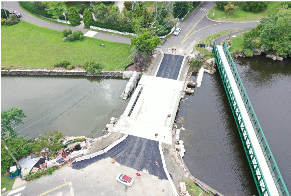
Aerial image of Davis Avenue Bridge on August 31, 2021.
